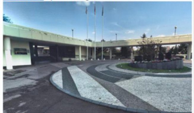
Location B Lower level, view from SE
